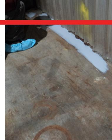
Belzona 5231 (SG Laminate) was applied by CMM's applicator, who was supported by the Belzona Technical Consultant. The product was applied with a short bristle brush along the edges and with a medium nap roller for all other areas in accordance with the Belzona Instructions For Use (IFU).
